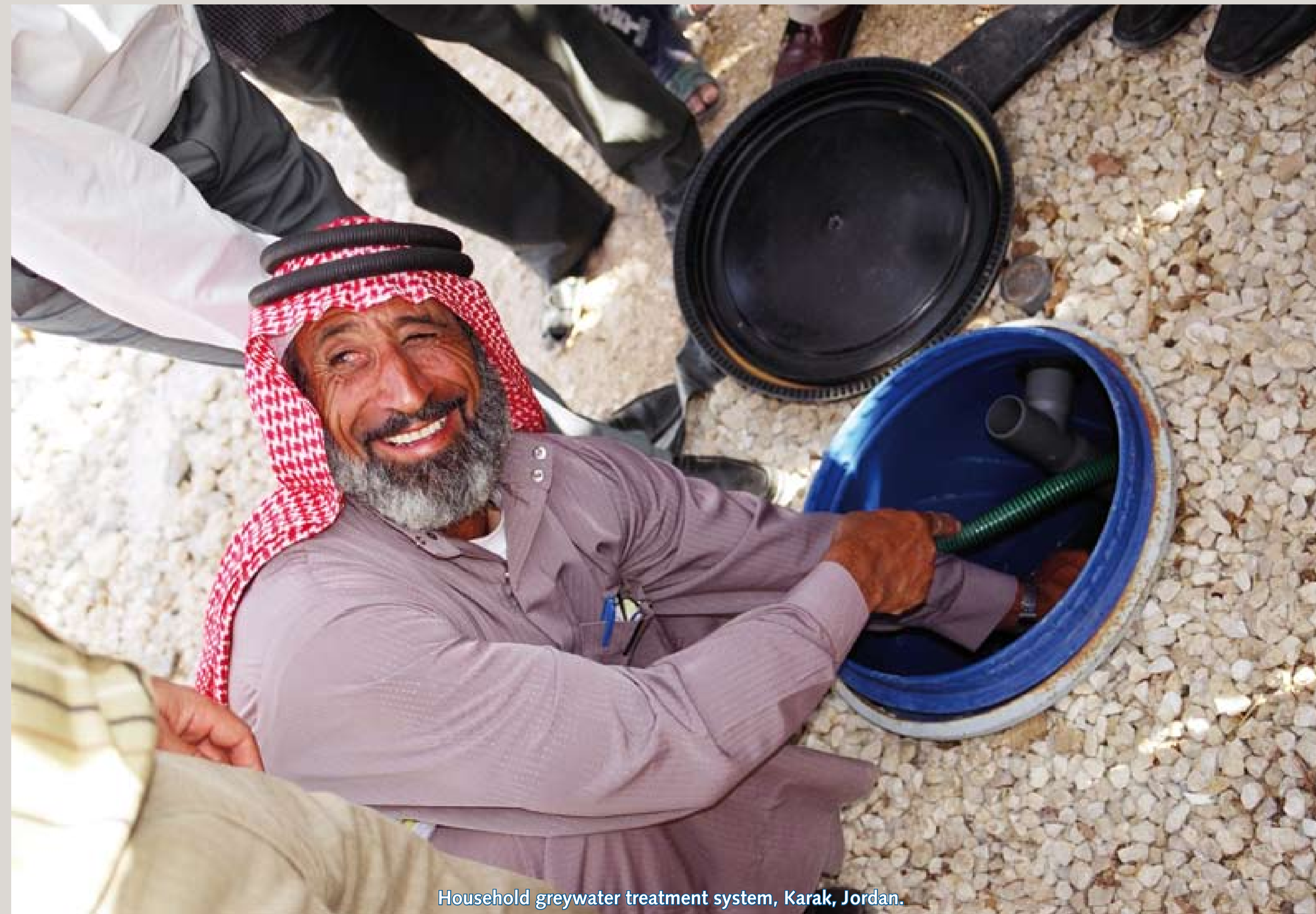
Household greywater treatment system, Karak, Jordan.
